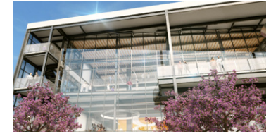
OUTDOOR PATIOS & BALCONIES
